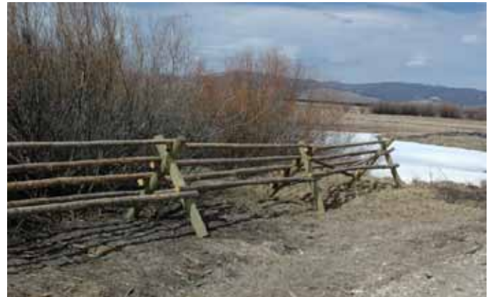
Recommended wildlife-friendly jack fence along a riparian area.
