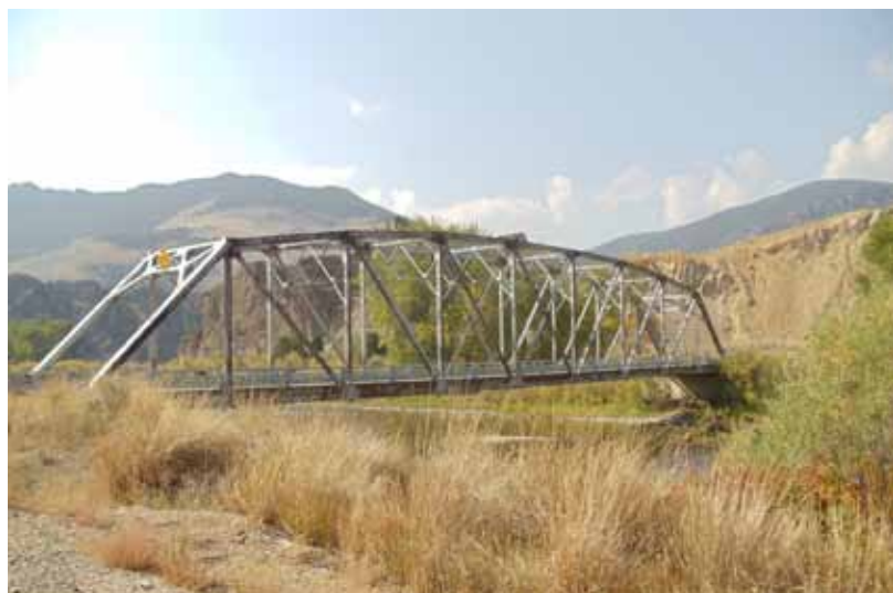
Existing bridge at Maidenrock. New bridges are subject to ordinances
