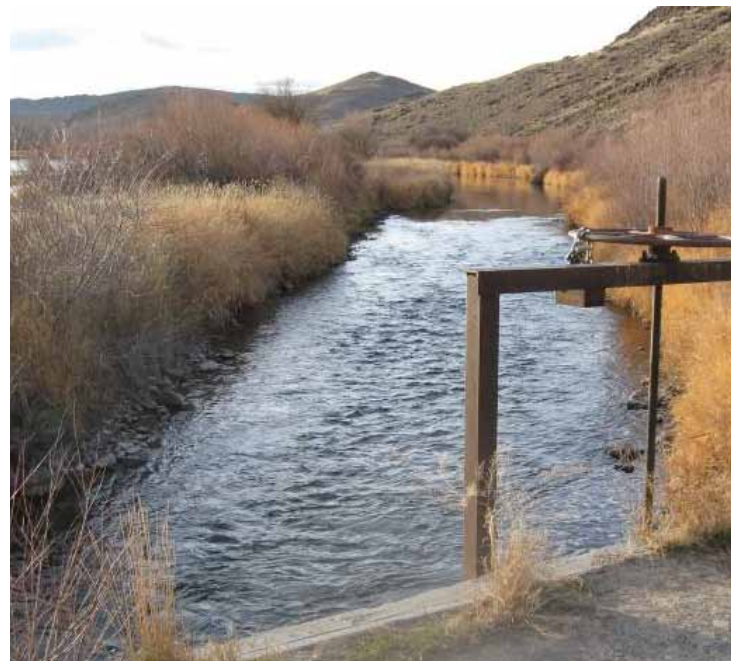
Irrigation ditch and headgate
