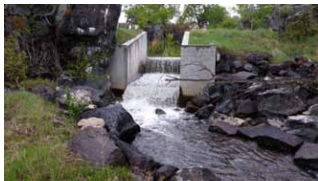
Fish barriers prevent nonnative trout from recolonizing upstream reaches, while allowing westslope to emigrate downstream. Photo of current Cherry Creek barrier courtesy of MTFWP.
